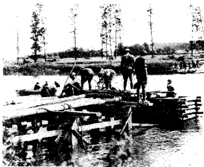
Soldiers of the 6th Engineers, 3d Division, build a trestle-crib bridge over the Marne River at Mézy (Aisne), east of Château-Thierry, France,
