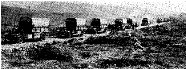
Another view of road constructed by 4th Engrs night before attack. Used 4,000 sand bags in it.
