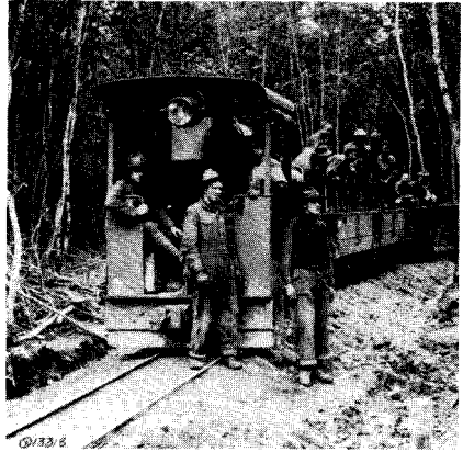
Engineers work on a narrow-gauge railway built to carry supplies to field artillery positions.
