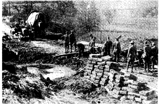
Another view of road constructed by 4th Engrs night before attack. Used 4,000 sand bags in it.
